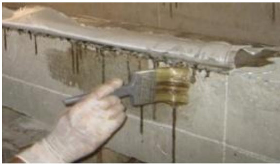
Figure: Application of epoxy and hardener on beam
