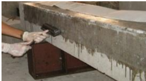
Figure: Roller used for removal of air bubbles
