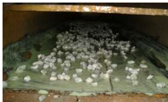
Figure: Application of epoxy and M-sand particles
