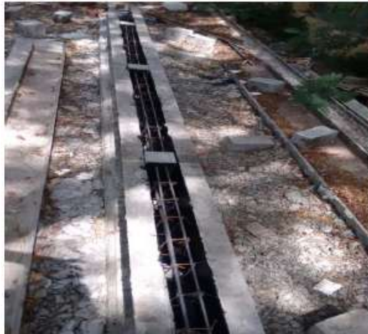
Fig: Moulds for casting beams
