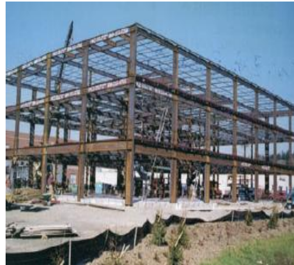
Pre-Engineered Building under construction
