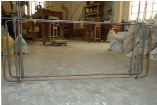
Figure: Reinforcement cage
