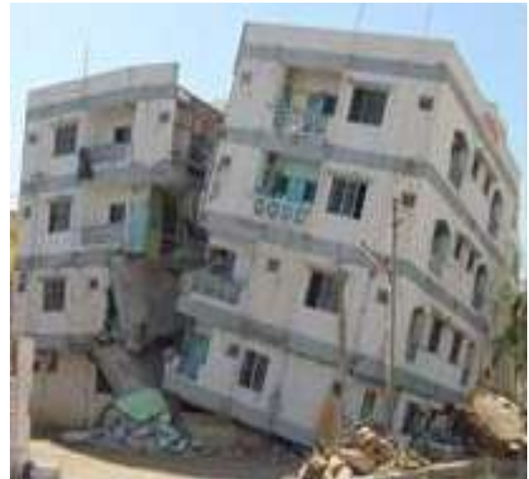
FIGURE 1.7 TOTAL HORIZONTAL EARTHQUAKE FORCE IN A BUILDING INCREASES DOWNWARDS ALONG ITS HEIGHT.
