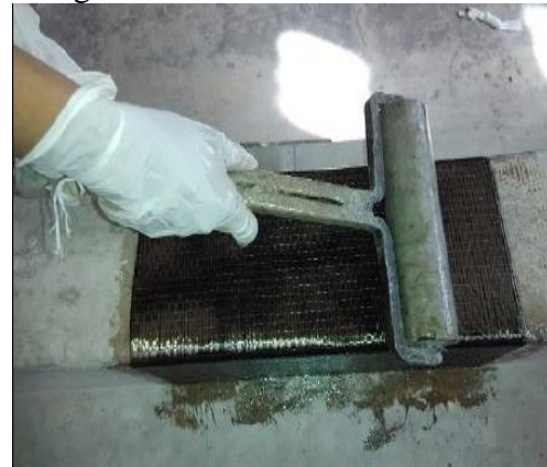
Roller used for the removal of air bubble
