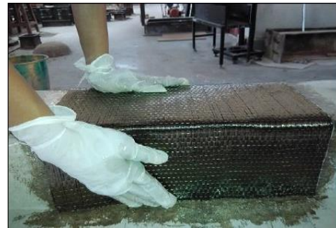
Fixing of BFRP sheets on the beam
