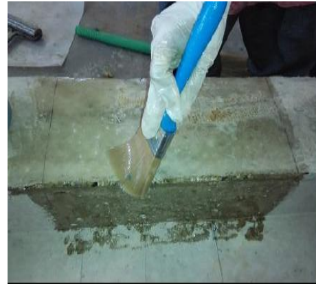
Application of epoxy and hardener on the beam
