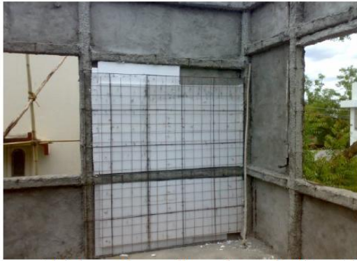
Shell house inside construction
