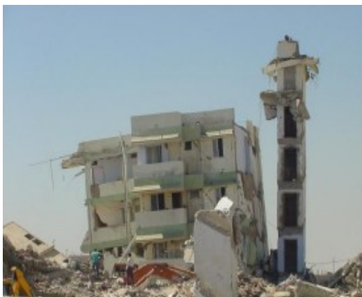
FIGURE 1.1 Collapse of RC Building Due To Insufficient Lateral Stiffness
