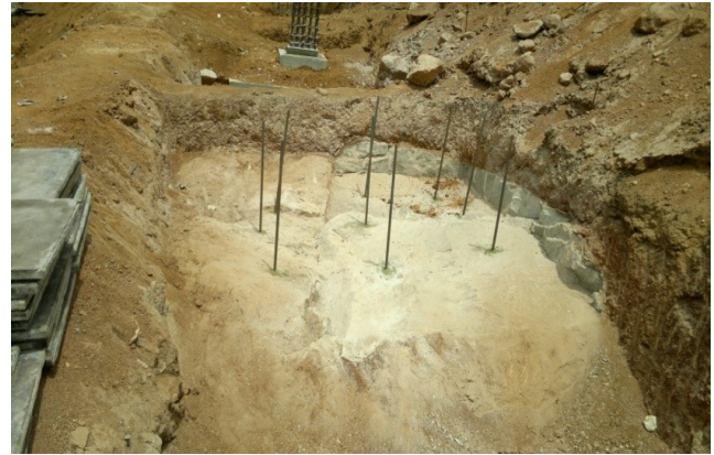
Fig.5.21:On site fixing of Dowel bars.
