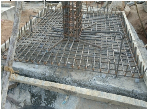
Fig.5.12:On site provision of mat.
