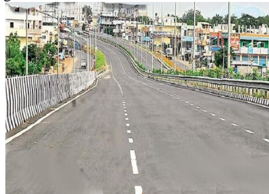
Narketpally Bypass 6 lane VUP at Khamam-Suryapet Junction
