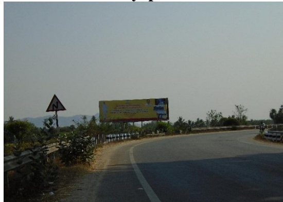
No Road Markings Sharp curve
