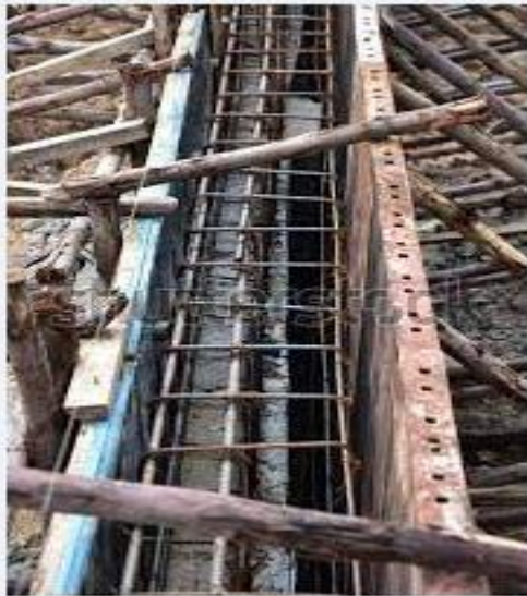
Figure: Casting of beam
